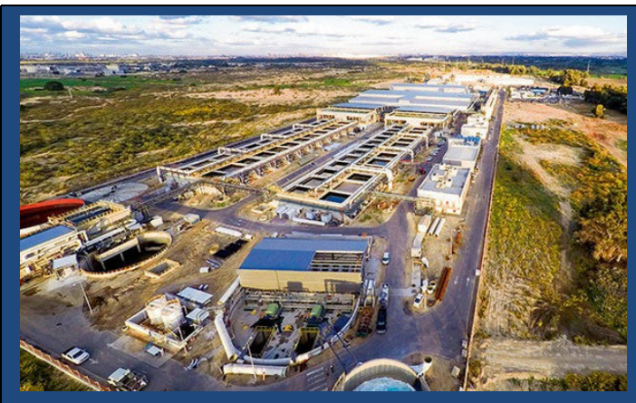
An Israeli desalination plant at Sorek
